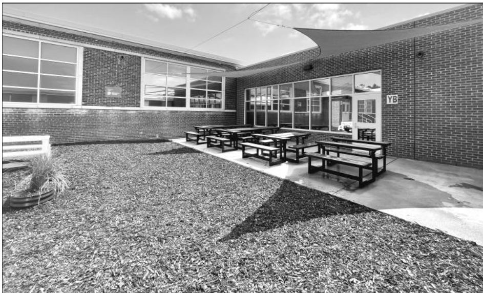
Completed outdoor classroom
